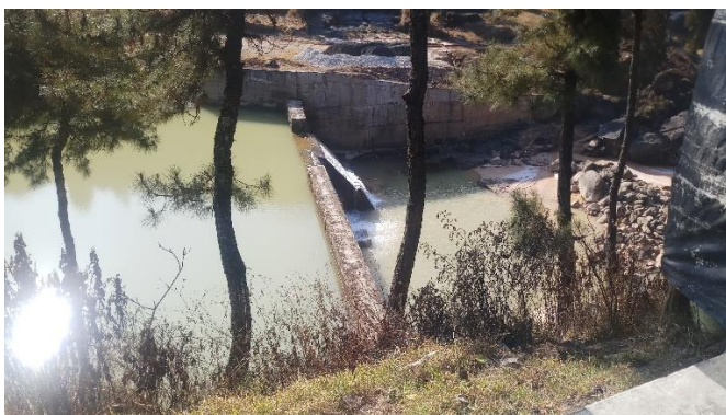
Figure 23 Silt filled silt trap in Umiew river in winters
