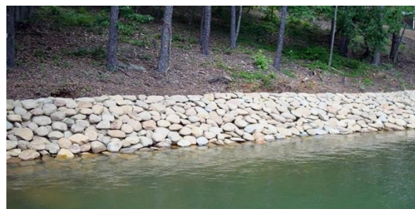
Figure 35 Stone retaining wall with plantations along the riverbank
