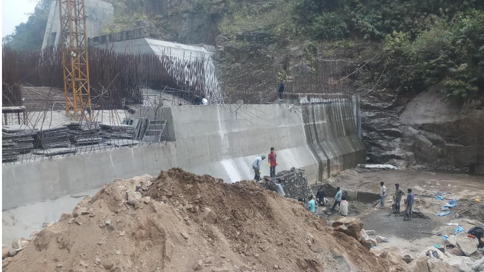
Figure 10 Hydro Power Project on Ganol catchment
