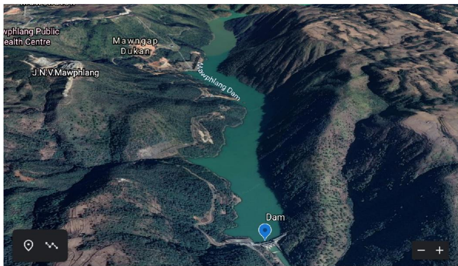
Figure 8 Mawphlang Dam - Greater Shillong Water Supply Project
